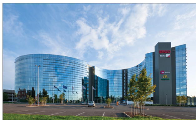
• Tammsaare Business Centre, an innovative office building on Tammsaare Road, Mustamäe.
